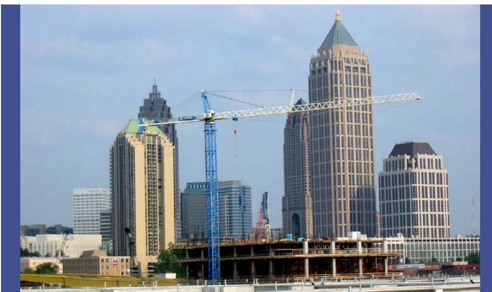
The Midtown skyline rises above the 171 17th Street construction site.
